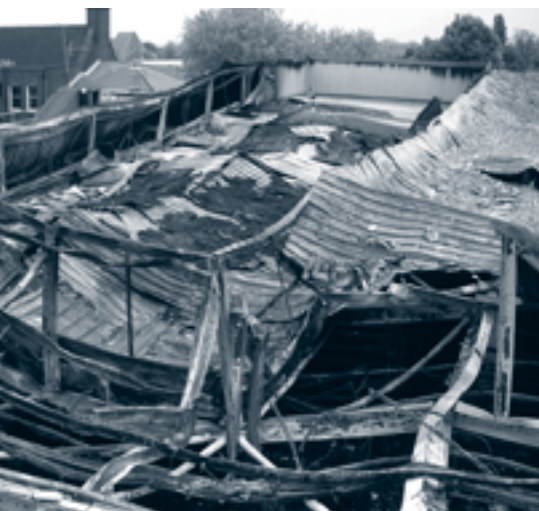
▲ PICTURE OF FIRE DAMAGED ROOF
