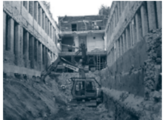
▲ FLOORS DEMOLISHED AND LEVELS REDUCED
